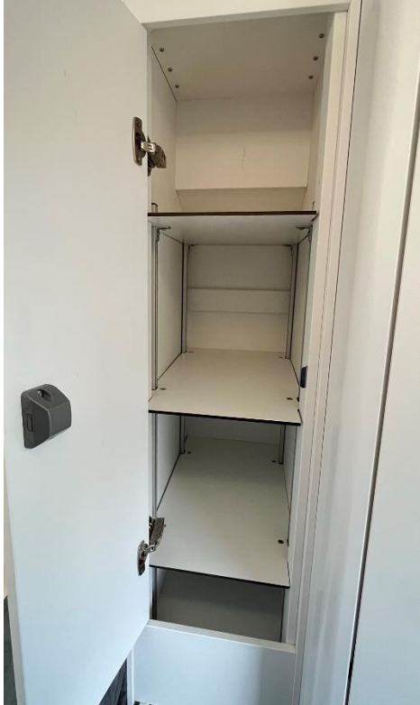
Figure 5. Positioning of aluminium tracks and shelves.
